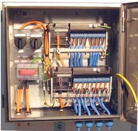
Intrinsically safe fieldbus barriers from R. Stahl allow connection of up to 16 FOUNDATION fieldbus devices per segment with half the footprint of conventional solutions. Units are designed to support typical current applications with up to 12 fieldbus devices and potential future implementations with up to 16 fieldbus devices.
