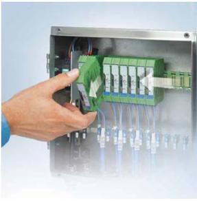
modular device couplers, FB-2SP or FB-ISO, based on hazardous area and isolation requirements, reducing installation costs by avoiding unused capacity and minimizing enclosure size. At the same time, a one-to-one coupler-to-instrument relationship increases operational integrity.
